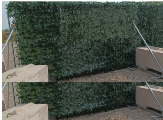
Plate 3.5 Heras fencing with attached textured plastic hedgerow (source: HS2/ EKFB, in Reason, P.F. and Wray, S. (2023). UK Bat Mitigation Guidelines: a guide to impact assessment, mitigation and compensation for developments affecting bats. Version 1.1. Charter
